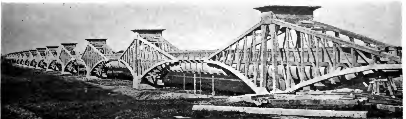
Cantilever Trusses and Cross Beams support oval pipe Reinforced-concrete construction throughout.
